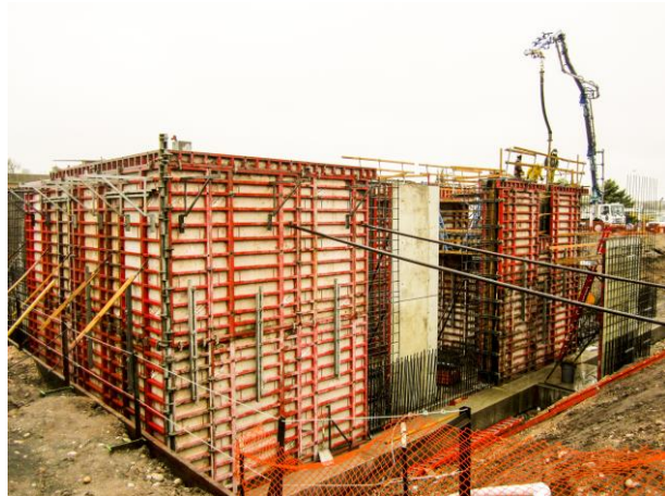
Construction of the DWRF South Process Train
